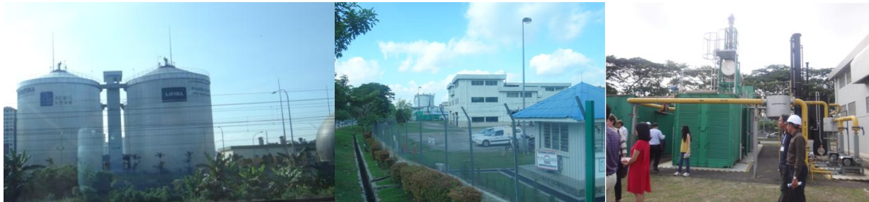
Top: IWK Sewage Treatment Plant, Pantai Dalam (top right: Biogas engine facility)
