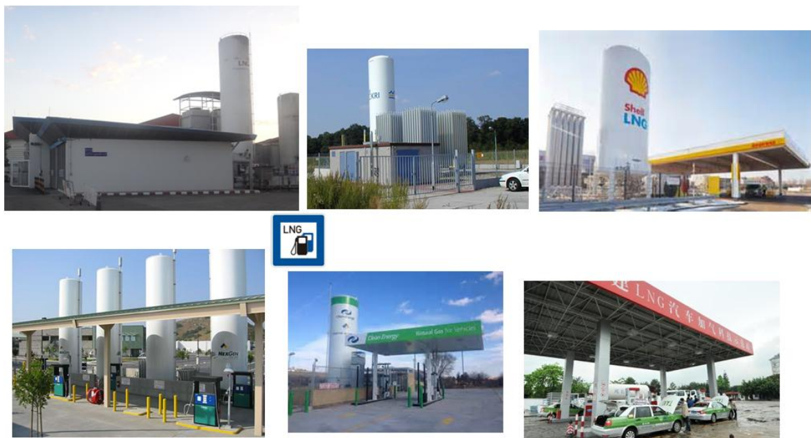
Figure 3: Examples of LNG and LCNG stations
